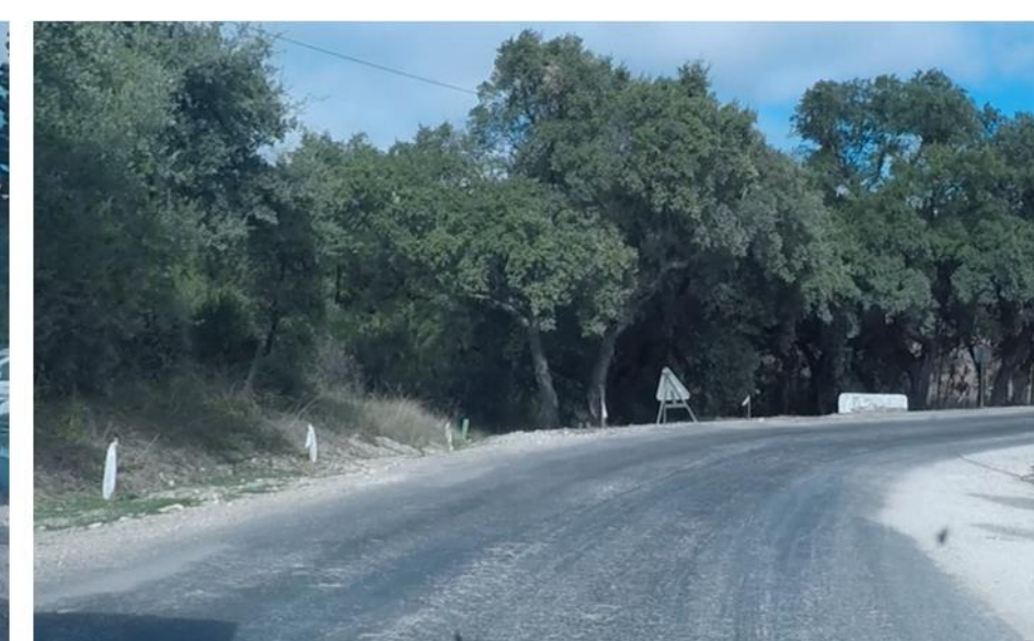
Specific areas of the recycled layer presenting some surface ravelling
