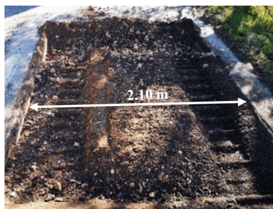
In situ extraction of reclaimed material
