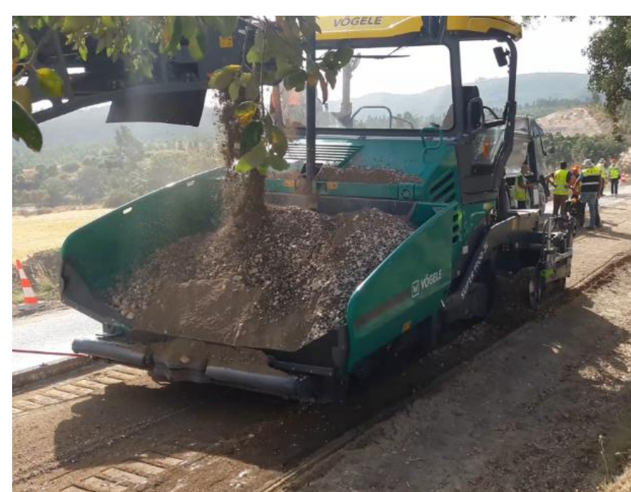
Paver used to apply the new recycled layer in the pavement trial
