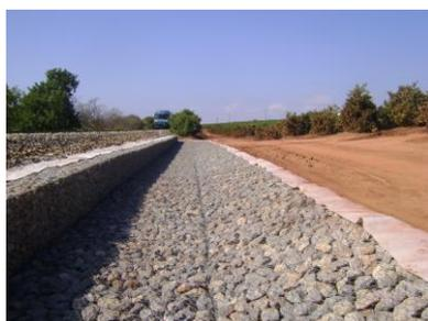
Actions developed with a view to stability, extension of the useful life and guaranteeing the safety of railway operation, under which the railway platform retaining wall was rehabilitated and reinforced, between km 388.395 and 388.560 of the Algarve Line, and an embankment stabilised with the extension of a gabion wall, between km 225.372 and 225.403 of the South Line.
