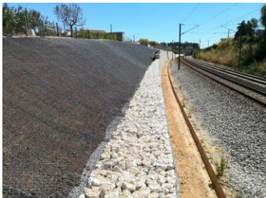
This intervention had the objective of improving the stability conditions of the excavation slope in the municipality of Soure, where there were several scars of landslides and ravines caused by erosion and water infiltration, guaranteeing the conditions of railway traffic in this section of track on which the maximum speed is 220 km/h.
