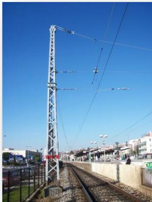
These works viewed to repair and paint overhead line posts in this railway line which is adjacent to the sea, and therefore exposed to significant deterioration and corrosion.
